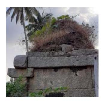
The Gopura, constructed of brick is in a much dilapidated state leading to the growth of Vegetation, that subsequently damages the stability of Shrine.
