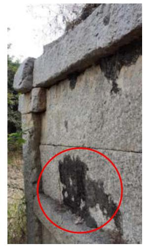
(Image on the left) Algal stains found on the exterior wall surfaces.
