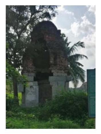
The brick Gopura is in a much dilapidated state leading to the growth of Vegetation, that damages the stability of Shrine. Though a part of the structure has got destructed, major portion of them are in a state that can be restored. Thereby, reconstructing the just the missing portion.
