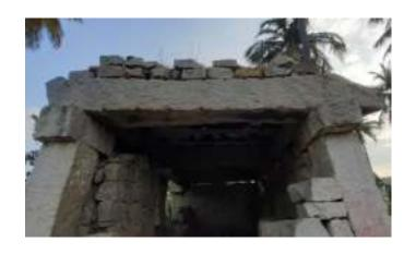
The stone masonry on the roof is in a dilapidated state leading to the growth of Vegetation. Care must be taken to remove the Vegetation and restore the roof structure, covering it with a damp-proof coat.
