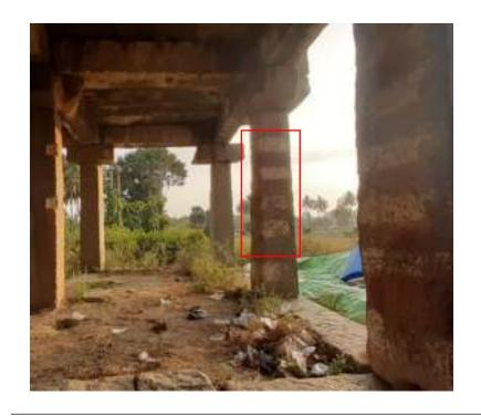
Pillars painted with white enamel bands to be removed as they degrade the integrity of the structure.
