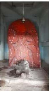
Sanctum gateway and main sculpture unsympathetically coated with enamel paints- degrading the integrity of the shrine and needs to be thoroughly removed.
