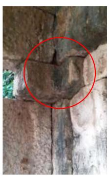
Dampness retaining on the wall surface and lack of maintenance has lead to the formation of moss over it. Core cleaning of the walls suggested to remove the algal stains post which the surface would be coated with a damp-proof layer.
