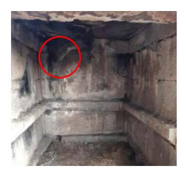
Dampness retaining on the wall surface due to poor indoor air quality and lack of maintenance has lead to the formation of moss over it.
