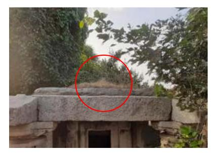
The stone masonry on the roof is in a much dilapidated state leading to the growth of Vegetation.
