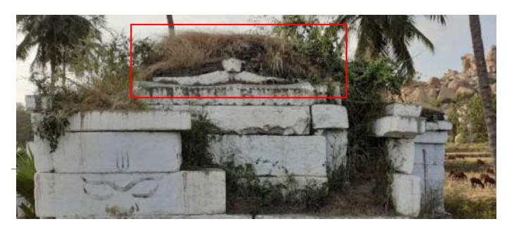
The Gopura, constructed of brick is in a much dilapidated state leading to the growth of Vegetation, that subsequently damages the stability of Shrine.
