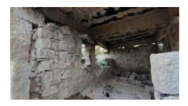
Spaces between the columns has been filled using stone masonry lately -that needs to be removed as it deteriorates the aesthetic significance of the shrine.
