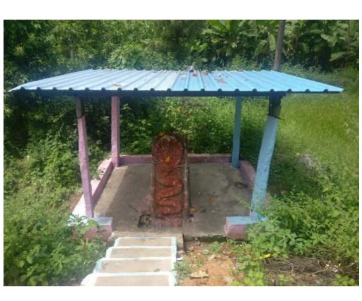
The structure over the Naga shrine has been constructed lately and the roof is unsympathetic to context. The asbestos sheet shall be replaced with an appropriate material that looks harmonious.
