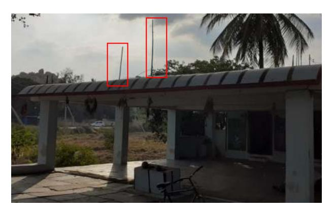
Steel bars projecting from the slab haphazardly that's been ignored since its construction.
