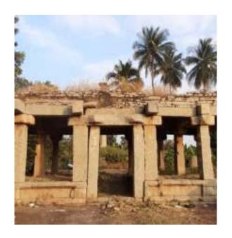
The stone masonry on the roof is in a much dilapidated state leading to the growth of Vegetation.
