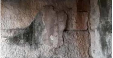
(Image above) Flaking of paint/ plaster added to the stone surface lately that has been affected with algal stains.
