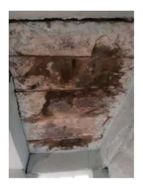
Patches indicating dampness is witnessed all over the ceiling that has penetrated from the roof.
