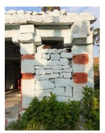
Spaces between the columns has been filled using stone masonry lately -that needs to be removed as it deteriorates the aesthetic significance of the shrine.
