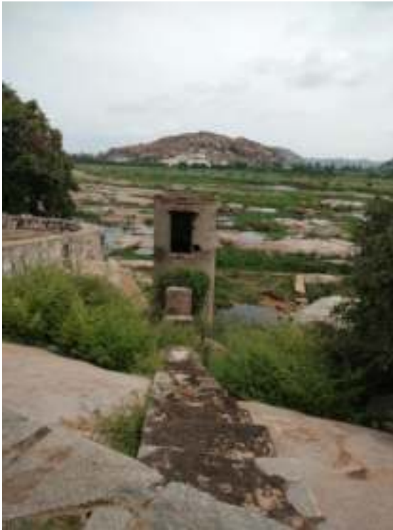
Figure 16: Water tank and steps to be removed.
