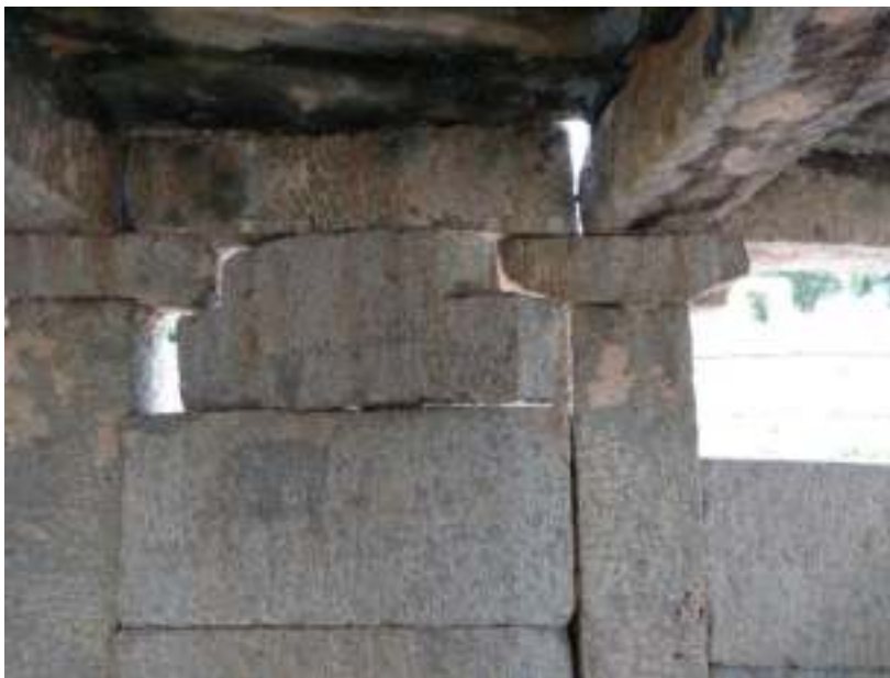
Figure 5: The granite blocks should be restored.
