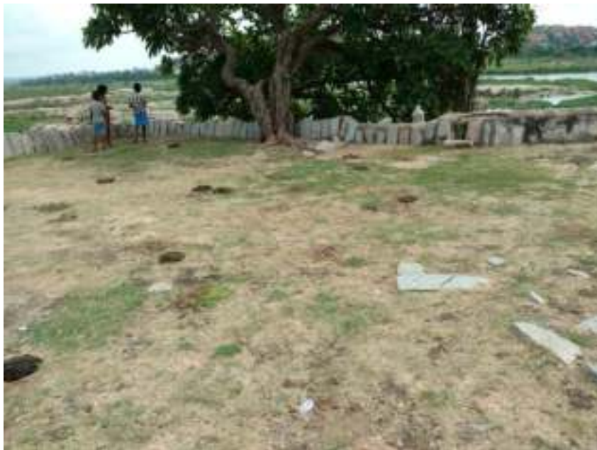
Figure 17: Courtyard at the entrance of the main temple should be levelled with compacted earth.
