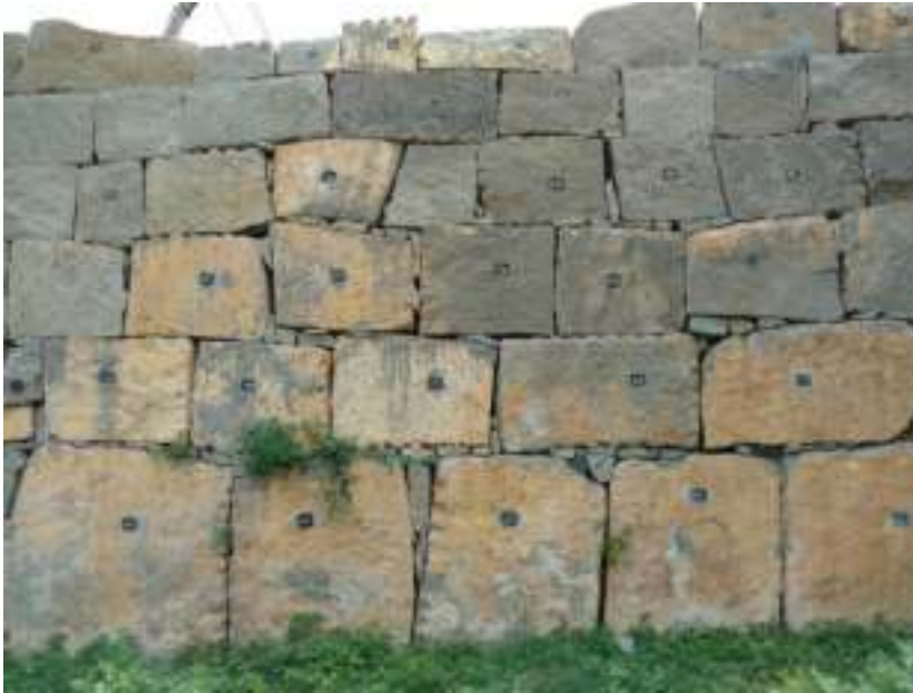
Figure 4: Numbering as seen on a wall near the North Gate at Aneundi should be avoided.
